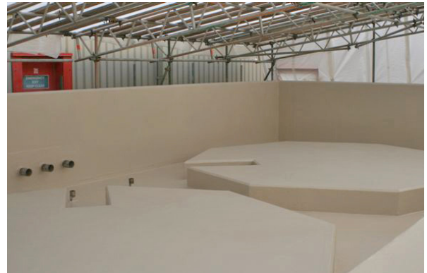
Coroflake lined concrete bund
